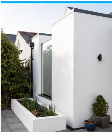
The double-glazed unit with a heat-soak treated toughened outer pane and laminated inner pane lowers emissivity, UV transmittance and noise pollution, helping to protect the new extension from external factors, without impacting the benefits of large glass panes.
